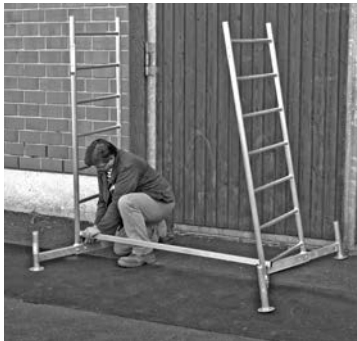
Basic scaffold with first extension
