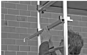
Basic scaffold with first and second extension
