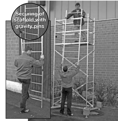
Basic scaffold with first and second extension
